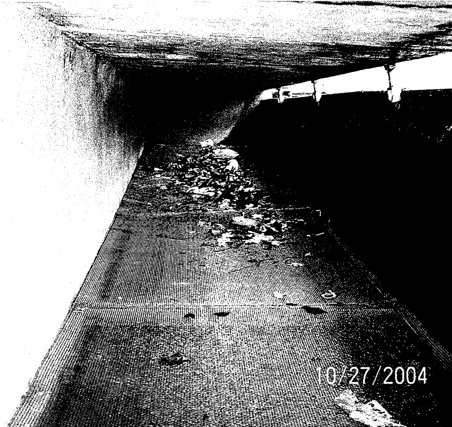
Figure 6 – Full Capture of Debris that Entered the Catch Basin
